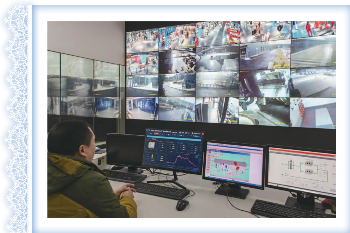
Employee in Changzhou monitoring the plant’s energy consumption and air conditioning operation
